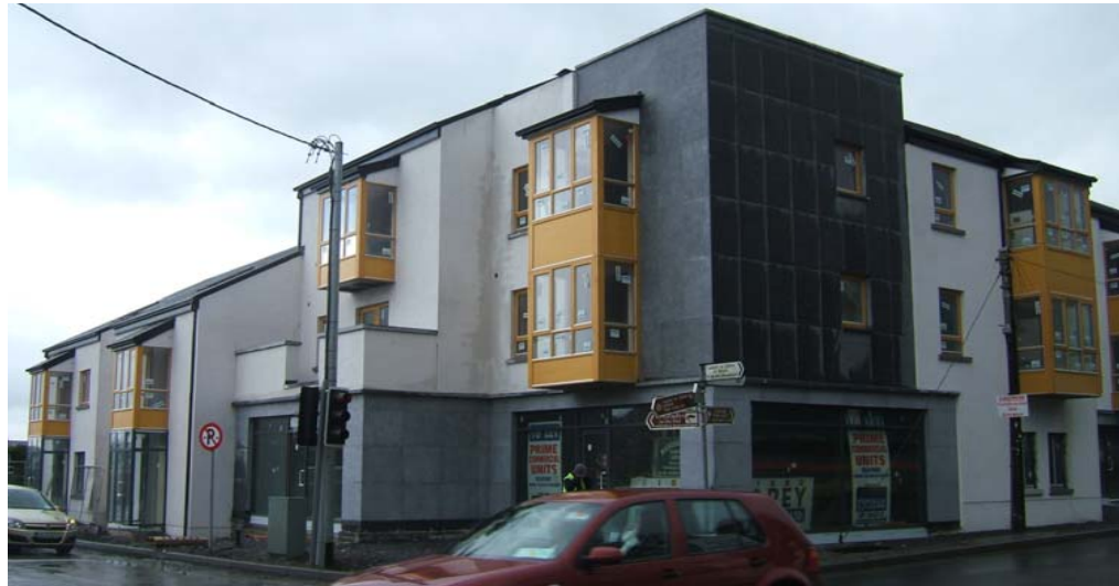
Pier Road/ R336 Corner
