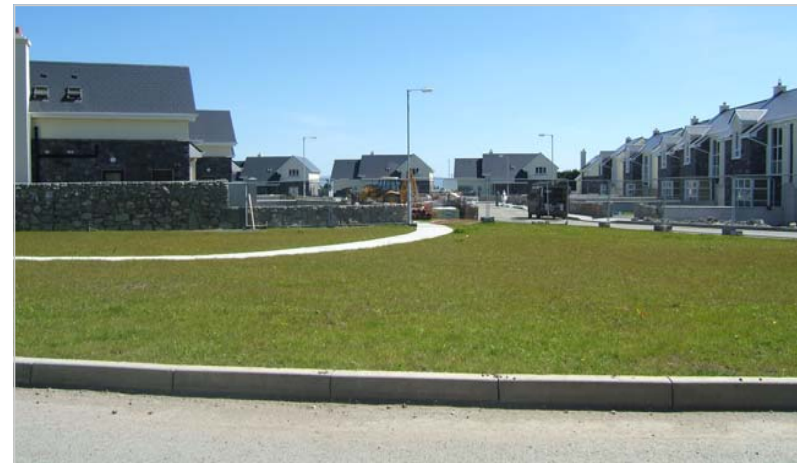
South facing view
