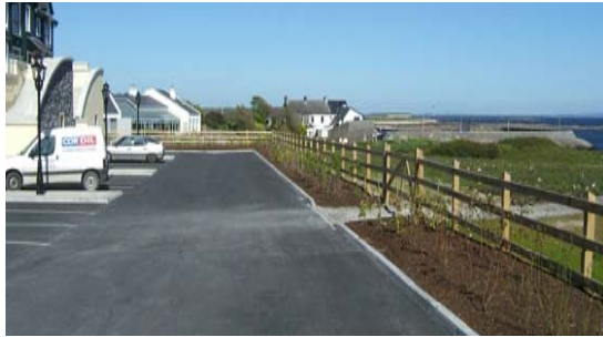
The above photograph shows the rear of Phase 3, including the access road, car parking provision and views over Galway Bay.
